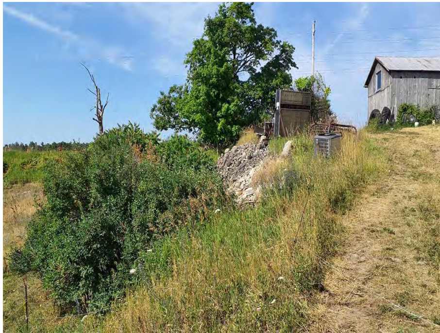
Image 3: Sloped area with example of gravel roadway disturbance encountered on site, facing southwest. 13 July 2022.
