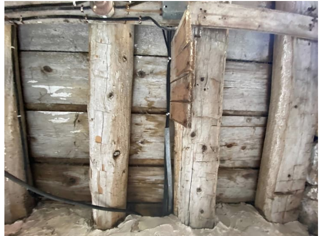
Plate 81: Hand hewn timber floor joists and wood plank subflooring
