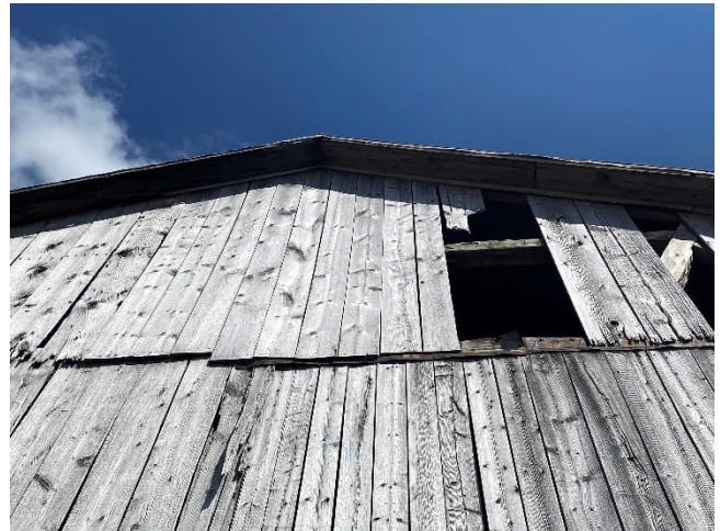
Plate 67: Vertical plank siding
