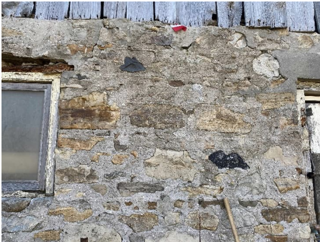
Plate 66: Granite fieldstone foundation with parging
