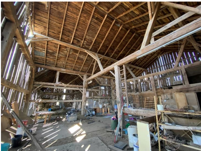
Plate 100: Timber framed post and beam construction
