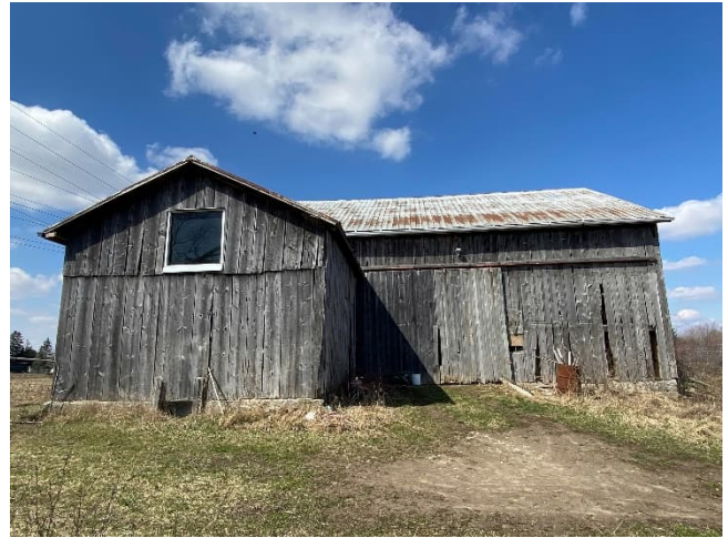
Plate 61: South elevation of the barn with banked earth access to loft
