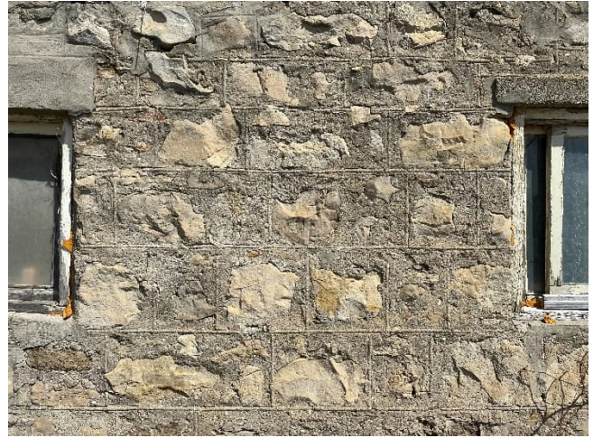
Plate 65: Roughly dressed stone foundation with scored parging
