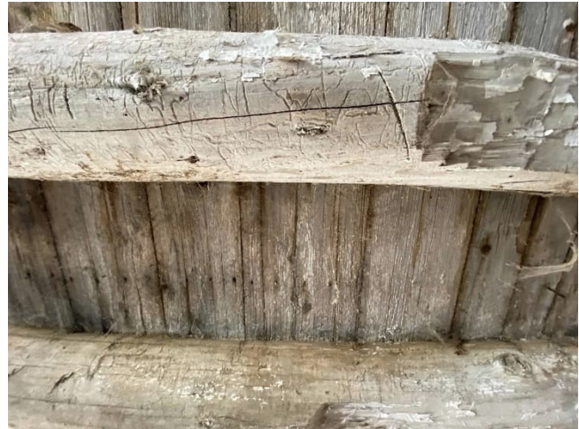
Plate 89: Timber left in the round used as floor joist
