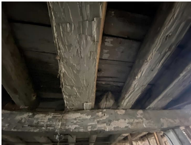
Plate 82: Hand hewn structural timber spanning the floor joists
