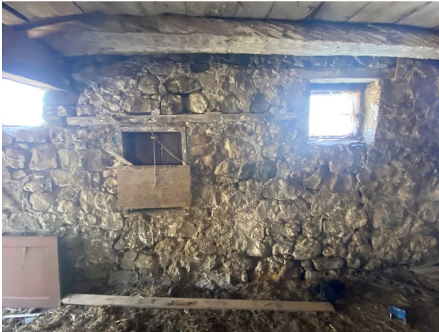
Plate 80: Stone wall with parging and inlaid bond timber course
