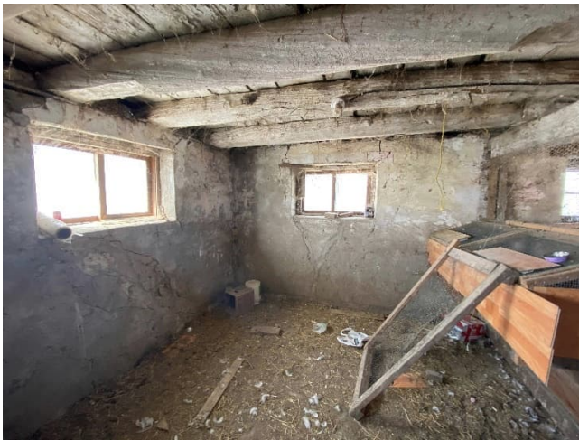
Plate 86: Northwest corner of north block
