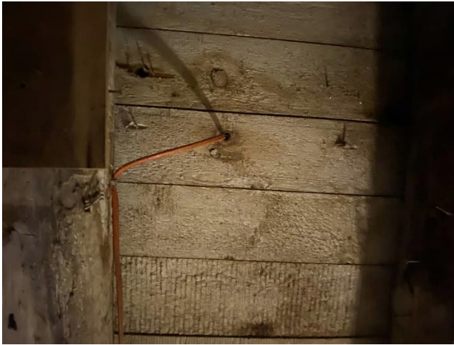
Plate 50: Dimensional cut wood plank subflooring
