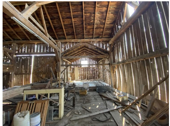
Plate 97: View south towards entrance door and drive floor
