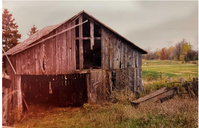
Plate 8: Mid-late 20th century photograph of the driveshed, since demolished (WCMA 2024f)
