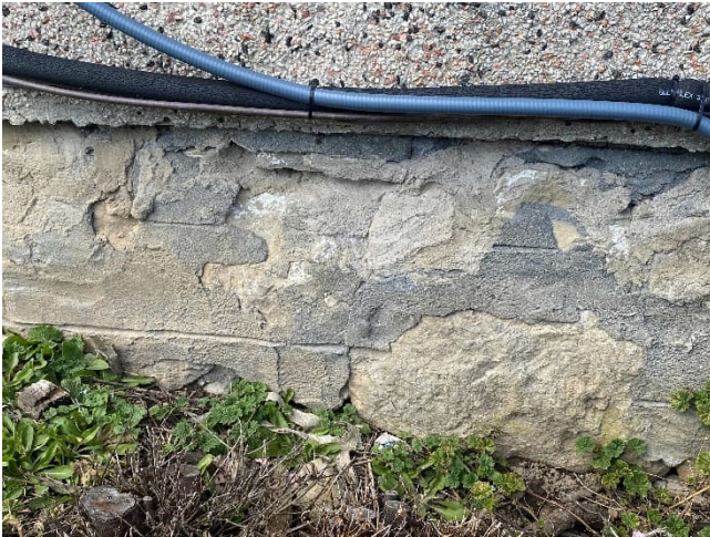
Plate 40: Stone foundation with scored parging
