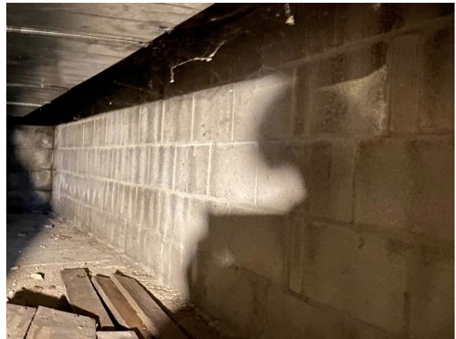
Plate 45: Concrete masonry units in basement crawlspace
