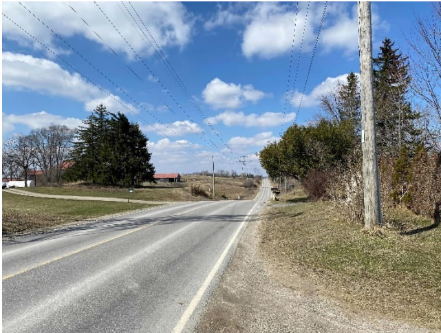
Plate 10: Looking North along Concession 7 from the Study Area
