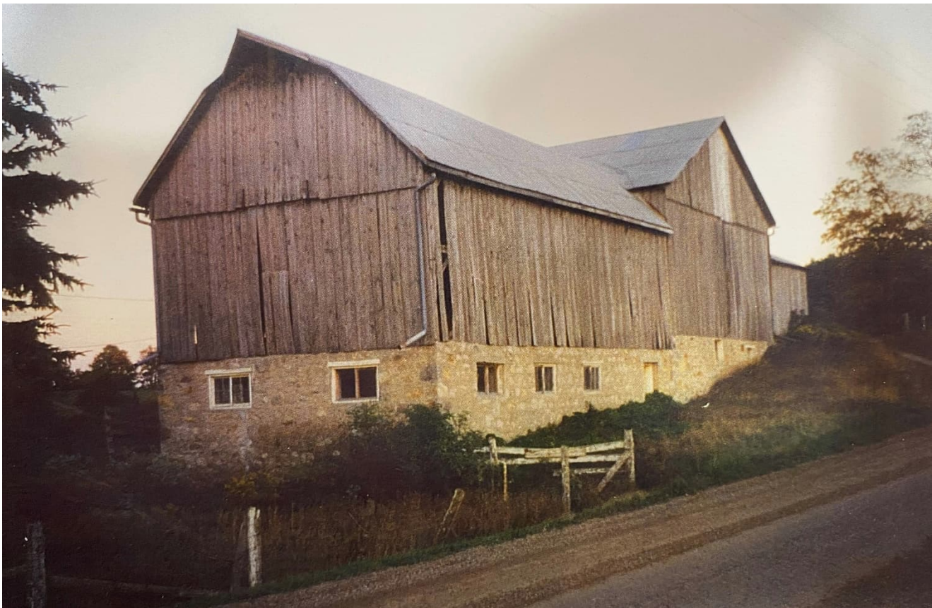
Plate 9: Mid-late 20th century photograph of the extant barn (WCMA 2024f)
