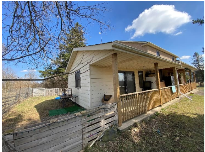
Plate 35: Oblique view showing the northwest elevation of the farmhouse
