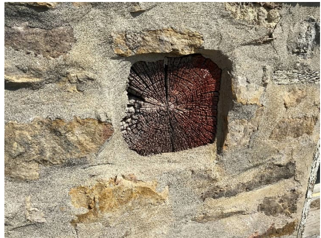
Plate 71: Structural timber laid into stone foundation
