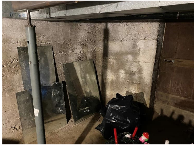
Plate 43: Poured concrete basement wall
