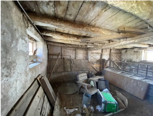
Plate 84: View south from entranceway into the north block
