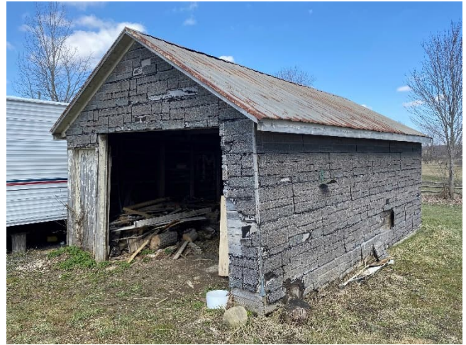
Plate 21: Wood frame outbuilding
