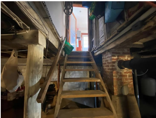
Plate 48: Stairwell to main floor
