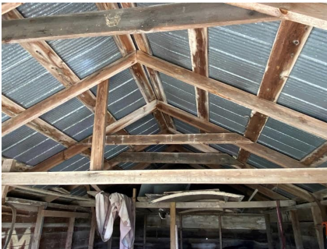
Plate 22: Interior framing of wood outbuilding
