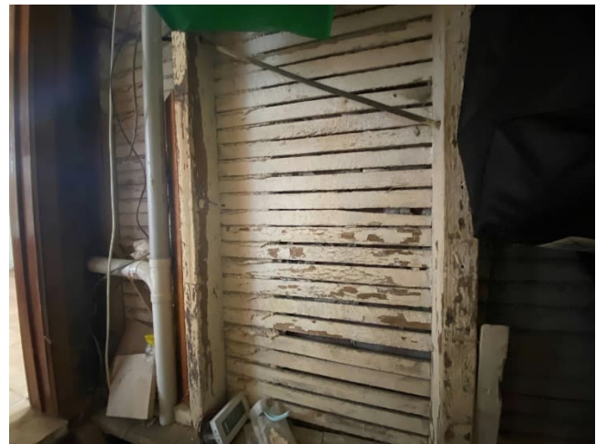
Plate 49: Lath and plaster finish within basement stairwell
