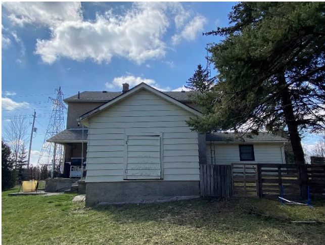
Plate 34: East elevation of the farmhouse
