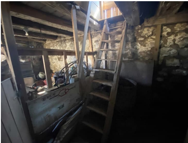
Plate 78: Access ladder from stable to barn loft
