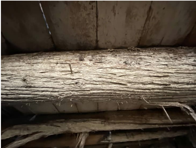
Plate 92: Whole timber floor joist
