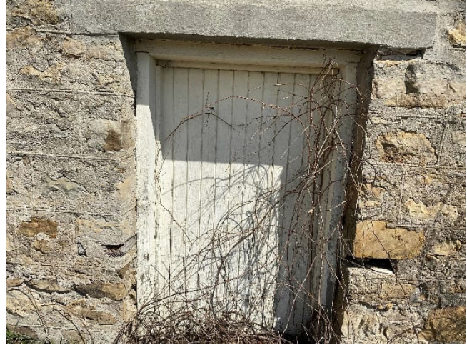
Plate 69: Wood door with concrete lintel
