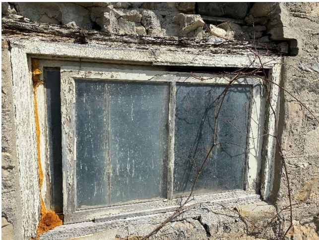
Plate 70: Window in foundation with wood frame
