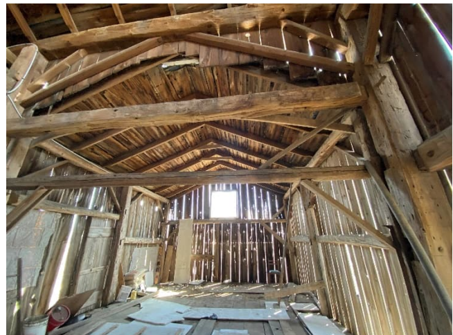
Plate 101: Vertical posts supporting bents, girts, and girt bracing
