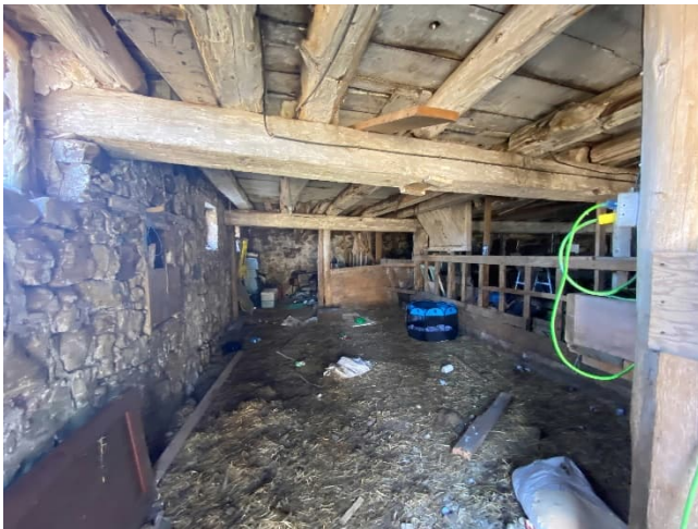
Plate 72: Looking south from the entranceway into the centre block
