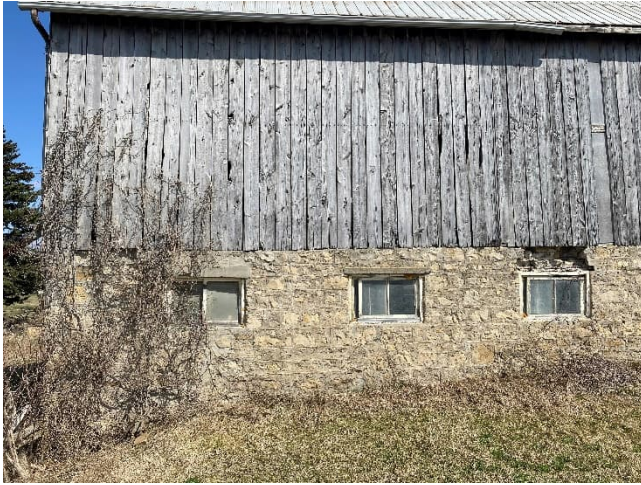
Plate 64: Stone foundation with fenestration
