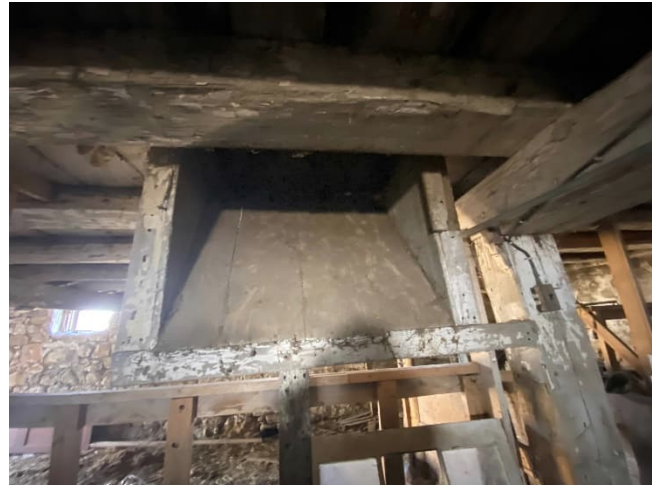
Plate 77: Feeding chute from upper-level loft into livestock stall
