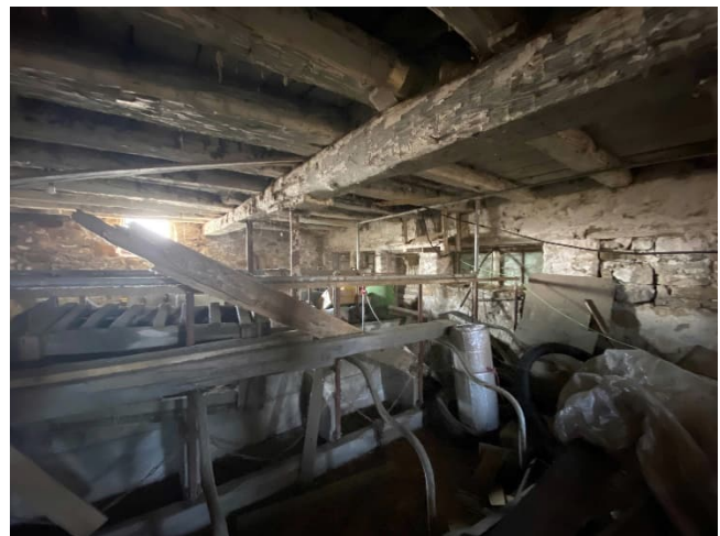
Plate 75: View of livestock stalls, looking northwest
