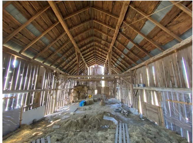
Plate 99: View north from the drive floor towards storage mow
