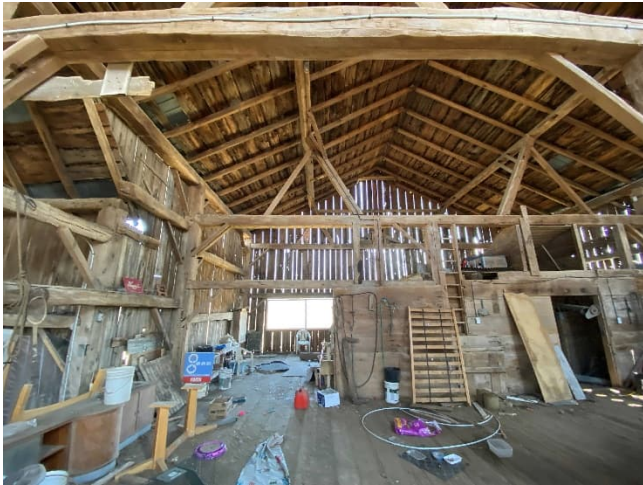
Plate 98: View east towards granary
