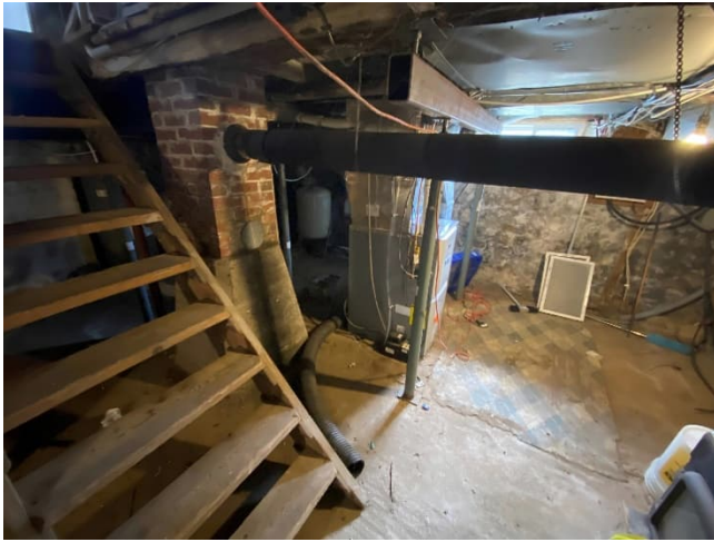
Plate 42: Central staircase and basement wall
