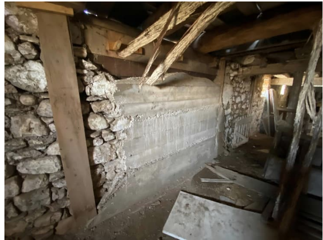
Plate 91: Section of south block foundation wall repaired with poured concrete
