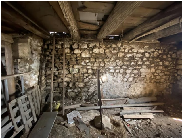
Plate 90: Rough stacked fieldstone foundation wall in south block
