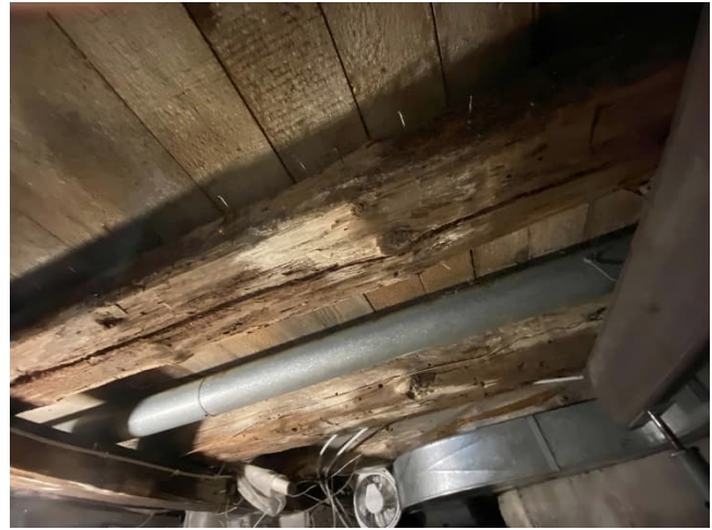
Plate 51: Hand hewn floor joists
